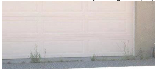
Don't let weeds occupy driveway cracks, giving your home an abandoned appearance and perhaps inviting suspicious activity.
