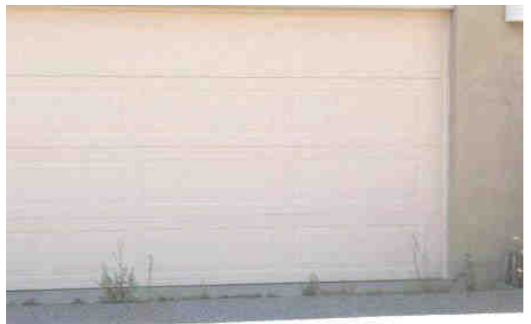
Let weeds occupy driveway cracks, giving your home an abandoned appearance and perhaps inviting suspicious activity.
